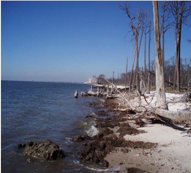
Figure 1: Deer Island Shoreline Erosion
